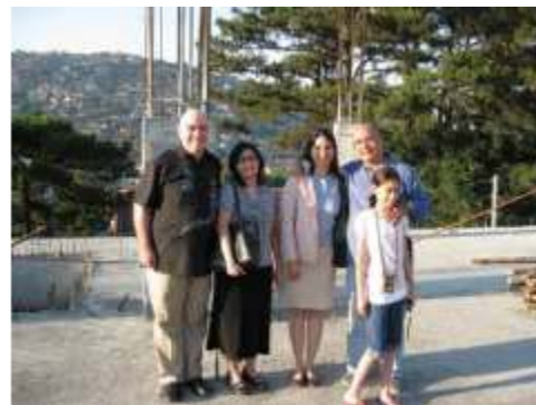
Beloved Ninong Pastor Robbie and Ninang Mavie Casas with their daughter Corinne at the construction site of the new GLCC building
